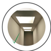
LIGHT WELL AREAWAY
